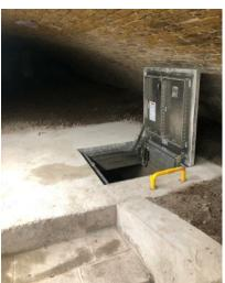
Because the Flip was located in the basement of a disused night club it was necessary to install an ATU 800 telemetry alarm which provides a remote alarm on failure to Thames Waters Control Centre at Maple Lodge which is manned 24/7.
